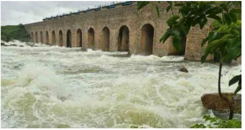
(FTL) of 1790.00 feet, holding 3.636 TMC of water. Authorities reported inflows of 1,800 cusecs and outflows of 2,630 cusecs, with six gates opened to two feet and four gates opened to three feet.
